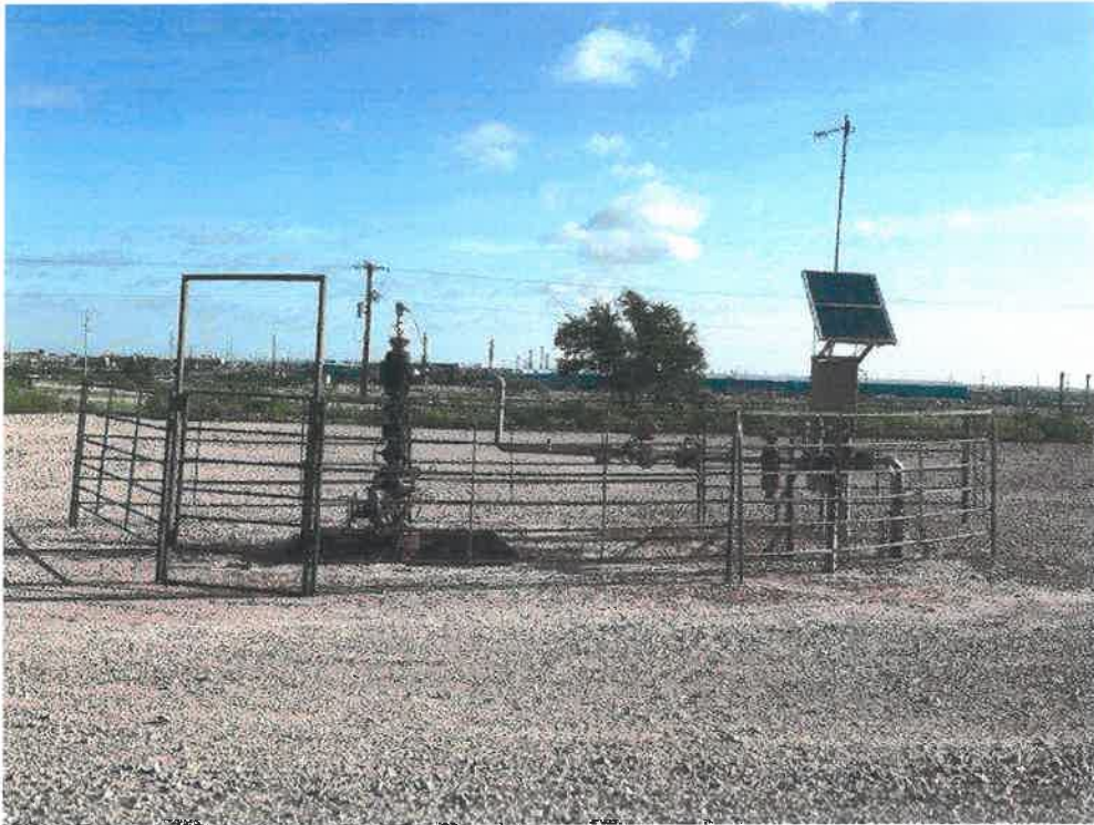
Photo 1. Typical fence panel currently at use at select SACROC well locations.
