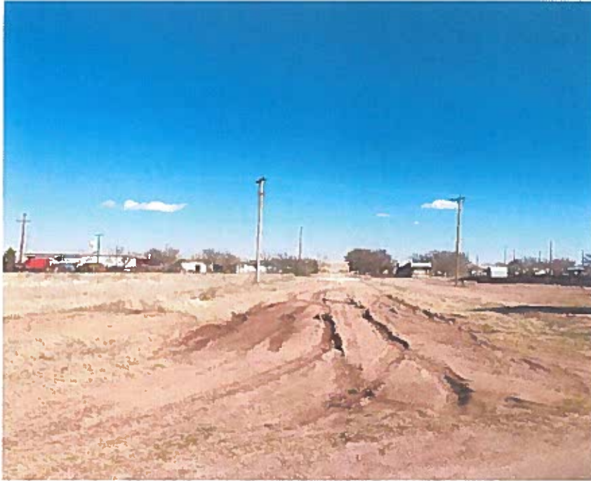
View from the west looking east
